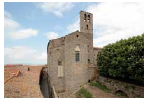
Church of S. Francesco, back façade
